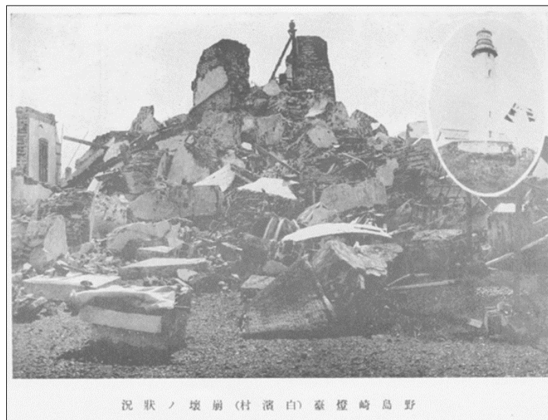
Figure 1. Collapsed rubble of Nojima-zaki lighthouse on uplifted strata in southern Chiba Prefecture (Source: Awa shinsai shi (Records of Earthquake Disaster in Awa Province, 1926)) https://tsunami-dl.jp/docimg/146/146_021.jpg/medium
