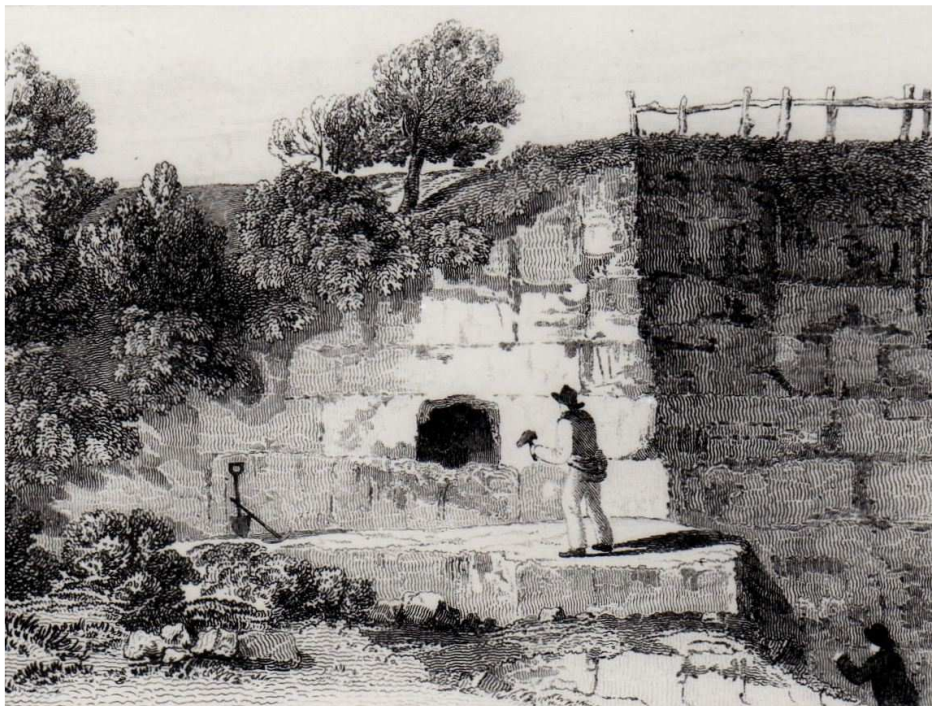
Fig. 1. The entrance to Kirkdale cave, as first exposed in 1821 by quarrying for building stone. Although lengthy, the cave was clearly much too narrow for mammoths and other large mammals to have been swept into it during the putative Deluge. Buckland argued that it had been a den of hyaenas, which had scavenged larger animals and dragged their dismembered carcasses into the cave, where their fossil bones were now found. (Author's collection)
